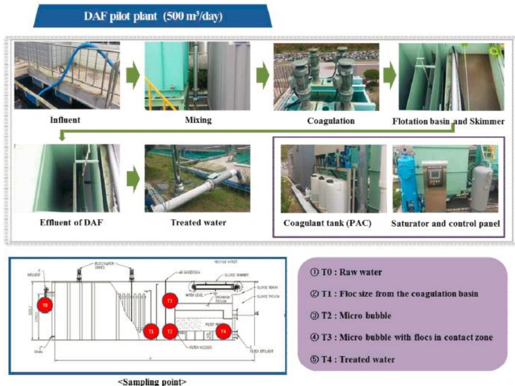
Fig. 2: Schematic design of DAF pilot plant (500 m 3 /d).
