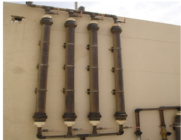
Figure.(2) Sand and activated charcoal filters.
