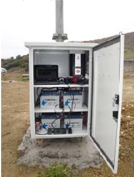
Figure 4. Charge controller, data recorder and deep cycle batteries.
