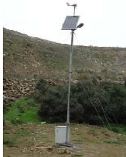
Figure 3. View of photovoltaic battery charging system .
