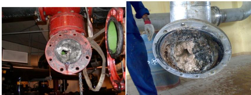
Fig. 1: Clogging of pipes by struvite at treatment plants
