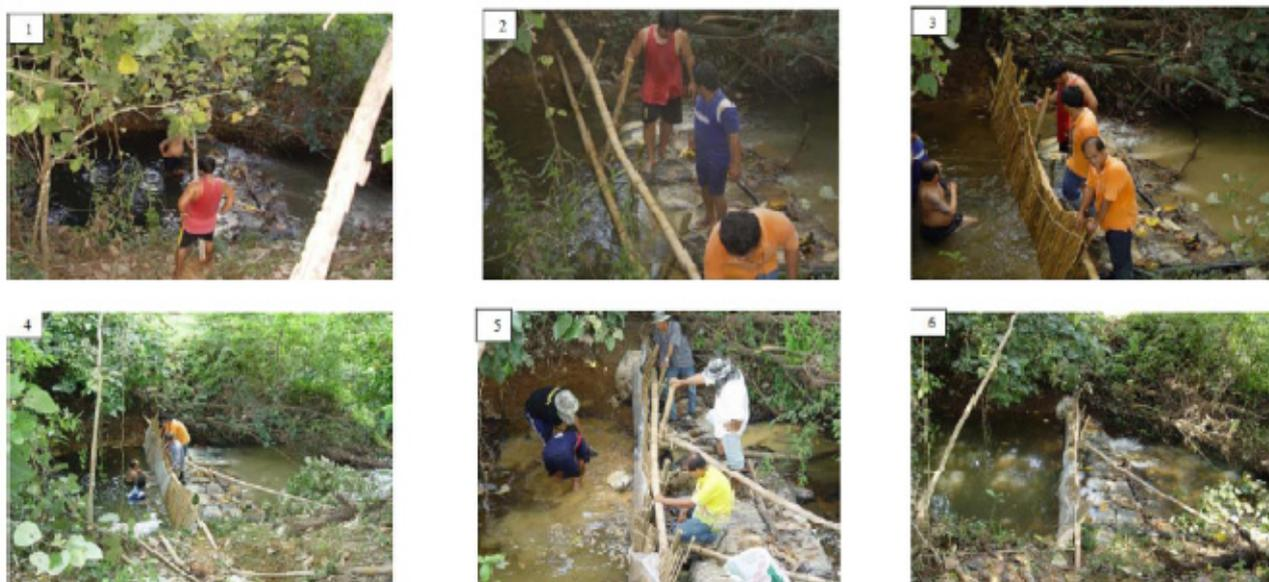
Fig. 1 Step of making low cost check dam with local material utilization following
